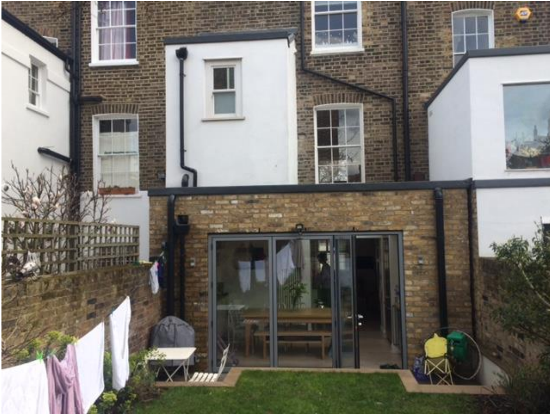
Image 1: View of rear elevation of the property
