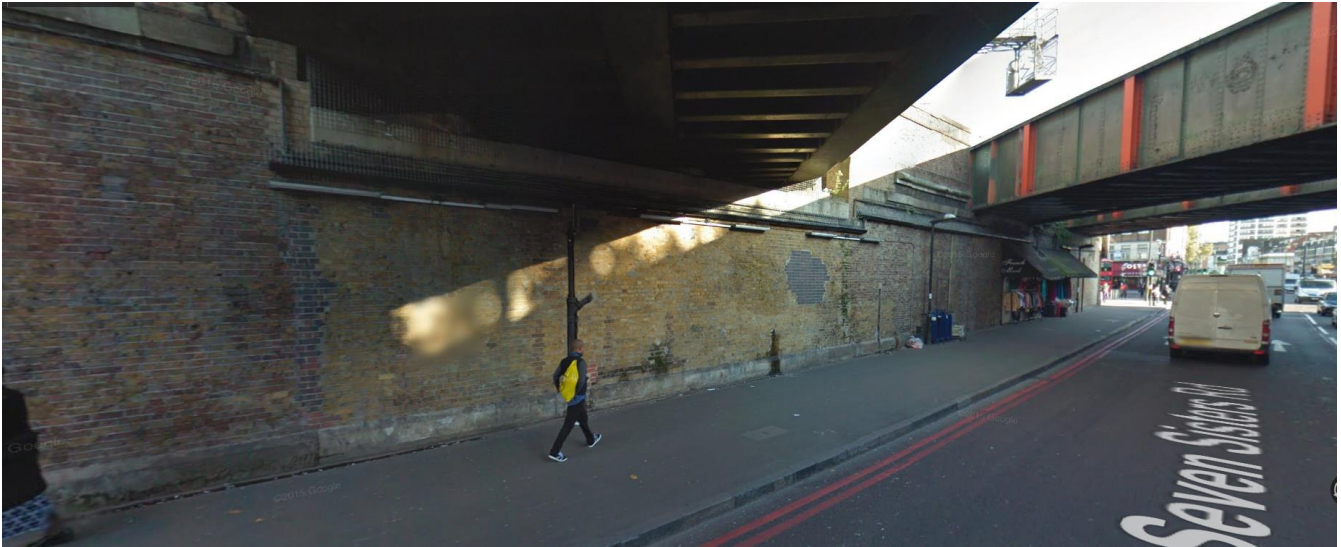
Image 2: View of northern abutments under bridges
