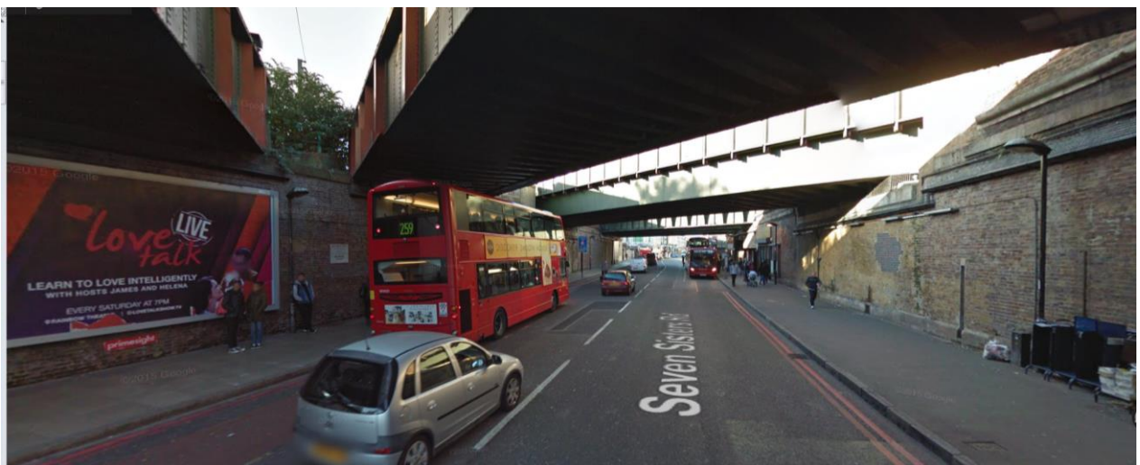
Image 1: View of area under bridges
