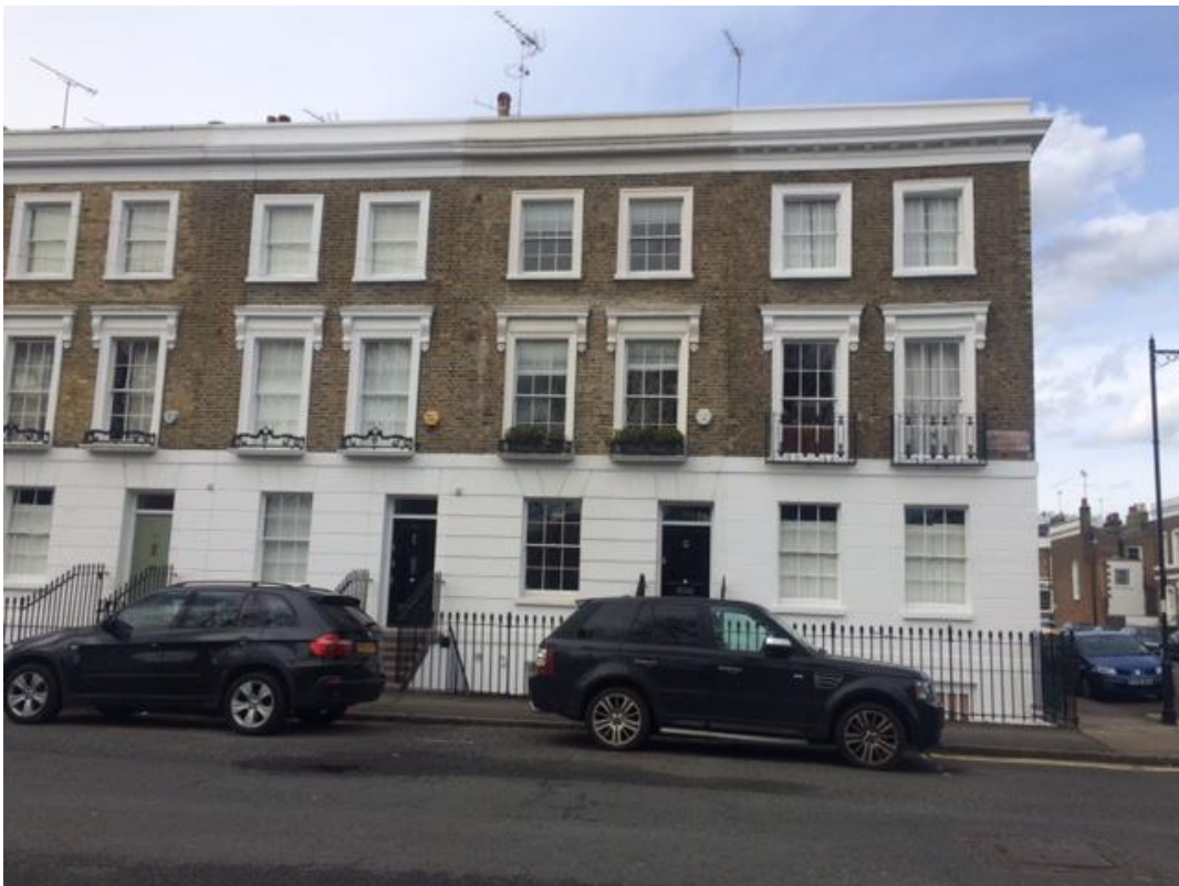
Image 2: View of front elevation of the terraced property
