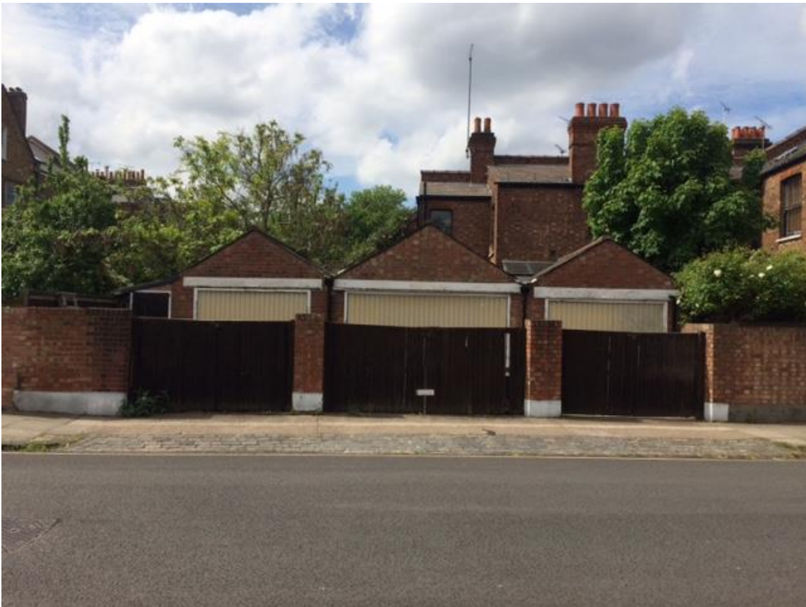
Image 1 - View of the existing garages from Quemerford Road
