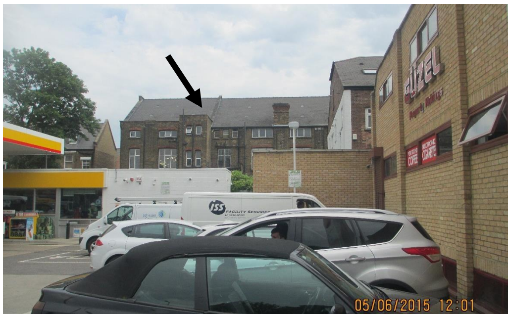
Image 3: Rear elevation of the site viewed across petrol station forecourt from Holloway Road.
